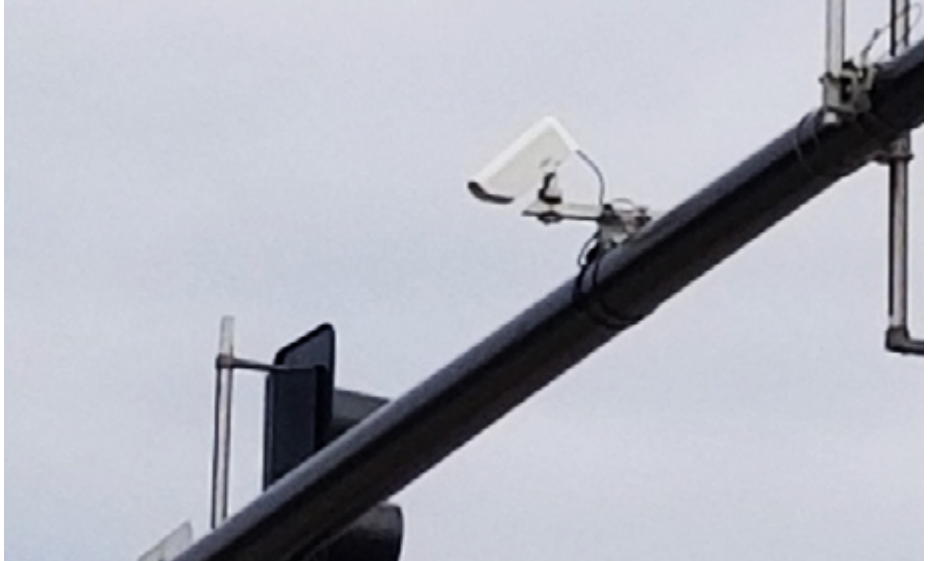
The IR Sensor mounted at an intersection in North Liberty, IA.
