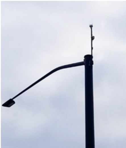
The Orion 533 weather station measures rainfall, wind speed and wind direction.
