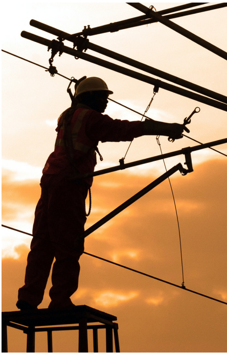
Monitoring weather conditions is critical to the safety of utility workers.
