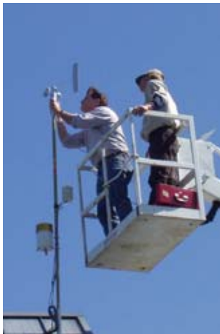
Jim Little, meteorologist for ODA, helps install the wind sensor at the Basket Slough National Wildlife Refuge.
