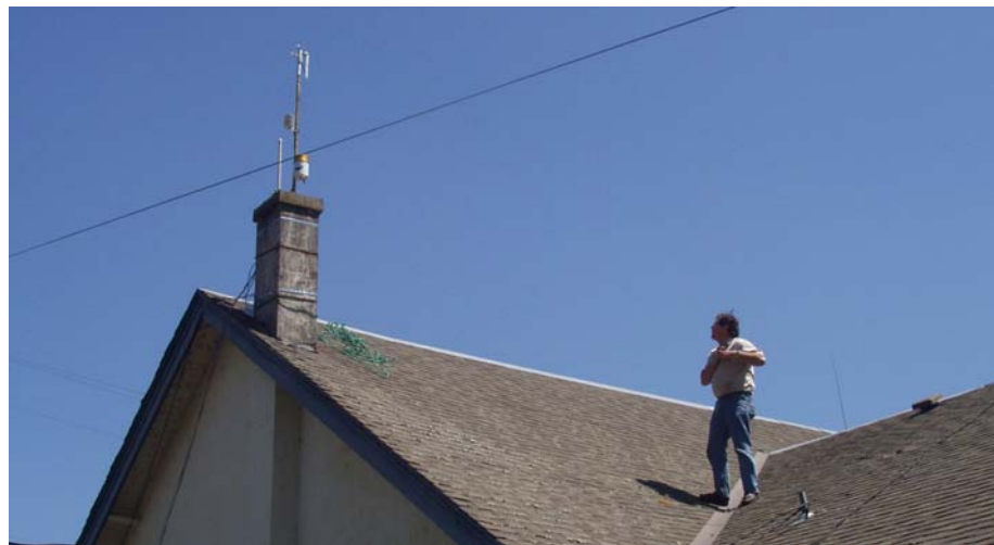
Jim Little checks the installation at Brownsville City Hall.
