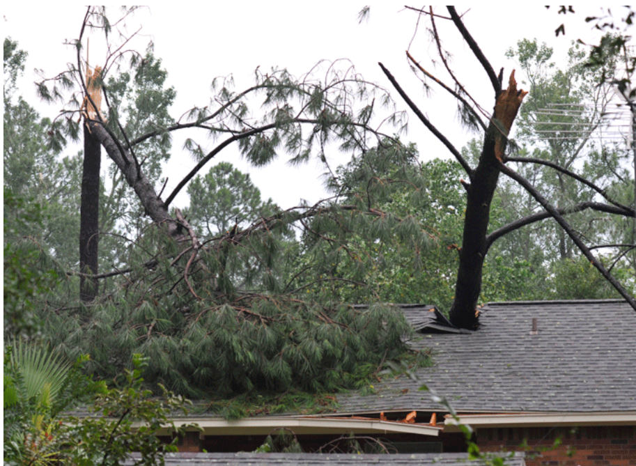
Falling trees made a hole in a neighbor's roof.
