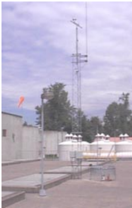
Wind sensors are mounted high over the waste water treatment facility.
