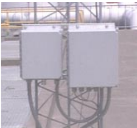
The control module and power supply are contained in weather-proof enclosures.
