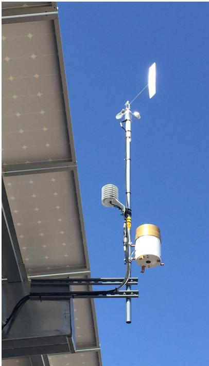
*Mounted on the carport: The Solar 2 Capricorn FLX Weather Station includes sensors for:*
